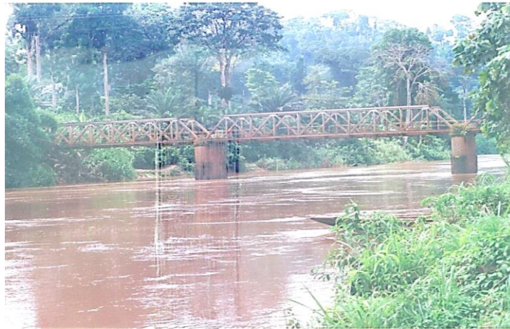
Figure 4: Northern Mongo Bridge at Etam-Kumba
