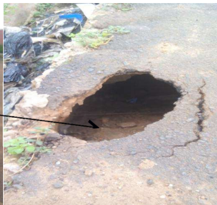
Plate 3: Partially collapsed Road at Alalawu area due to floods and waste blocking drainage.
