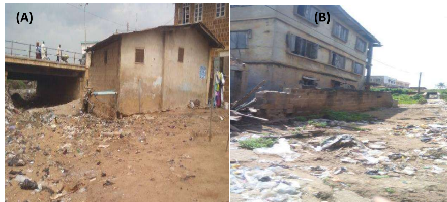
Plate 4: (A) Building located directly along a major water channel at Gada Aluko area a tributary of the River of Asa while (B) shows a building located on a flood channel at Mubo area.
