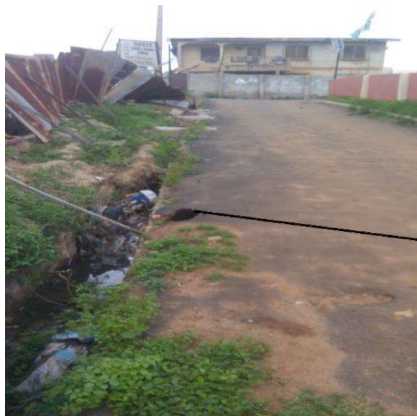
Plate 3: Partially collapsed Road at Alalawu area due to floods and waste blocking drainage.
